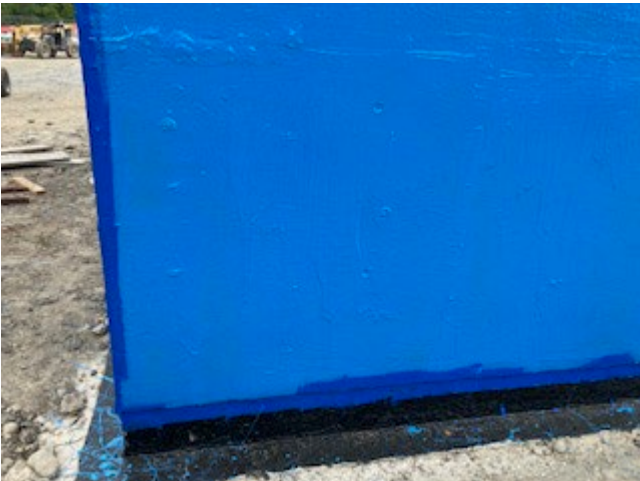
117 weather barrier application,
