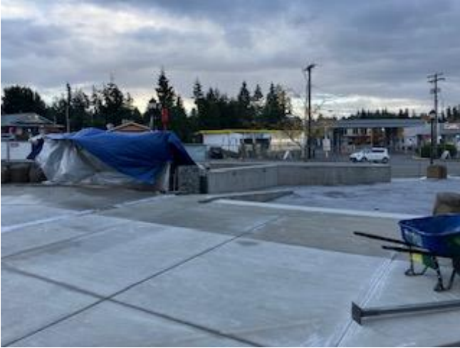
Station 111- Landscaping, fencing and Memorial plaza.
