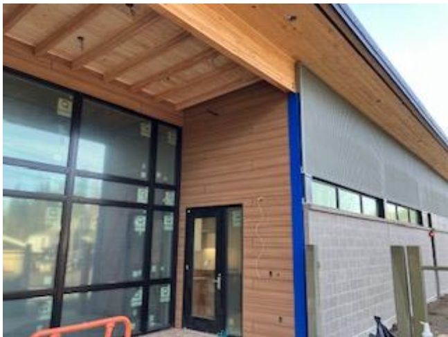
Siding is nearly complete.
