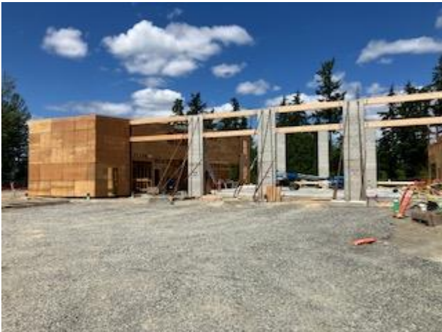
East and west side of the apparatus bay framing.
