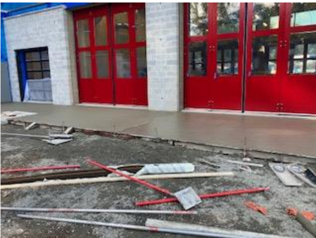
Concrete apron and sidewalks underway. Asphalt next week
