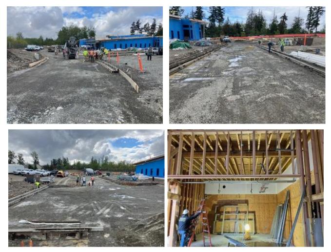
Interior framing nearly complete. Plumbing and electrical rough-in underway.
